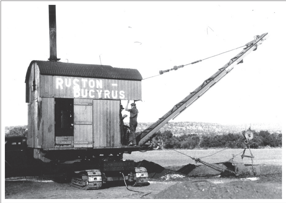
FIGURE 3.7: A steam shovel with dragline attachment, preparing a canal at the Marico-Bosveld project.
