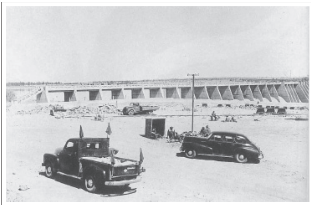
FIGURE 4.1: In 1950 the wall of the Vaal Dam was raised to secure a greater water capacity.
